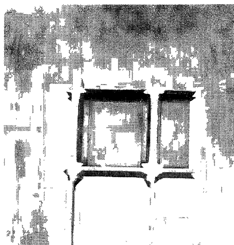
Photo 3. Forged diaphragm in panel zone section
