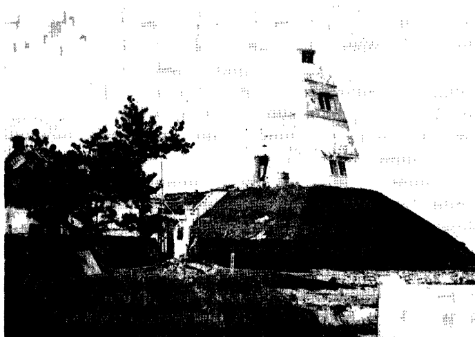
Photo 2 Lighthouse of Tenpozan in 1870 s 35) .
