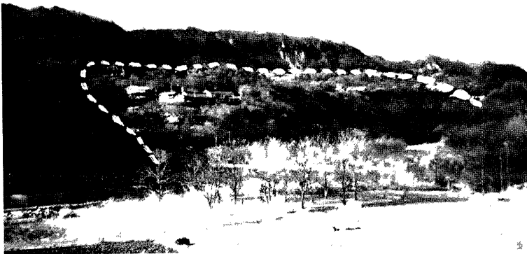
Photo. 4 The view of the Yamaura landslide taken from the opposite of Chikuma river (on the right side of the river). The enclosed part with the broken line showed the active landslide area.
