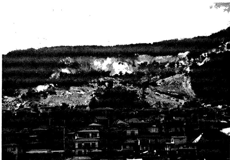
Photo. 8 The view of the Jizukiyama landslide taken from the Nagaono kindergarten in Nagano city on July 28, 1985. The front of the mudflows already had deposited in the Yuya house lot.
