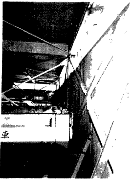
Photo 7 Buckling of steel braces
