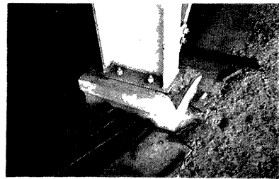
Photo 6 Damage at column base
