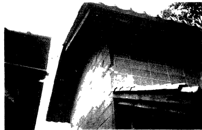
Photo 4 Cracks in concrete block wall
