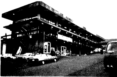
Photo 9 East annex of Kurayoshi city office building
