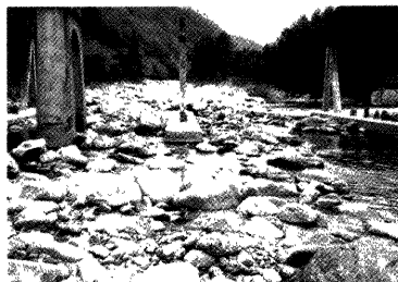
Photo. 1 Yokitogi Bridge looking upstream.
