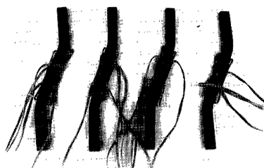
Photo. 3. Residual deformation of column A-Y after test.
