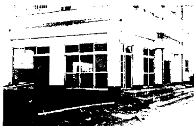
Photo. 18. Damage to glass panes in Tamina.
