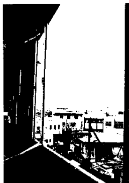
Photo. 19. Damage to glass panes of the gym.
