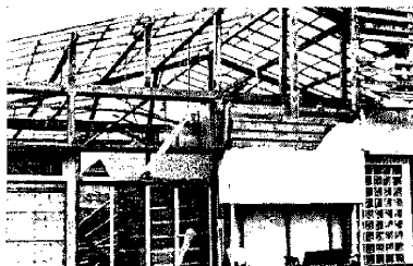
Photo. 3. A completely damaged house in Watomari.
