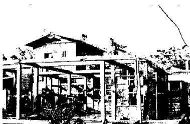
Photo. 5. A completely damaged house in Kuranuki.
