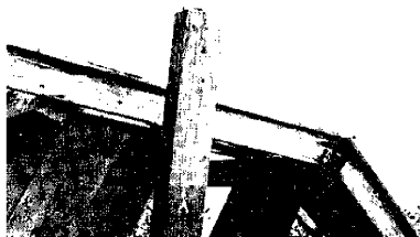
Photo. 8. Detail of a damaged beam and column.
