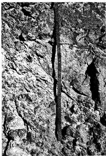
Photo. 7. Weathered sandstone in the landslide area.
