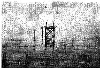
Photo. 1. Tower and poles for wave observation.
