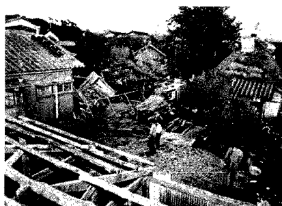
Photo. 3 Damage to structures.
