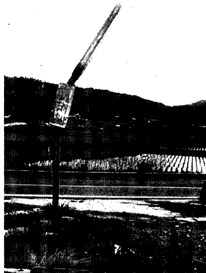
Photo. 7 Damage to the sign tower (2).
