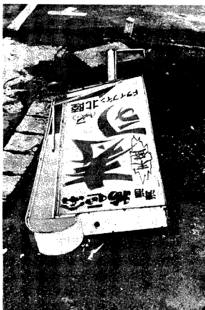
Photo. 6 Damage to the sign tower (1).
