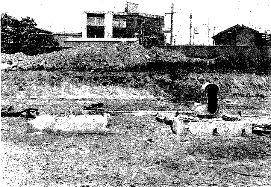
Photo. 2 Active (F2) and passive (F3) foundations
