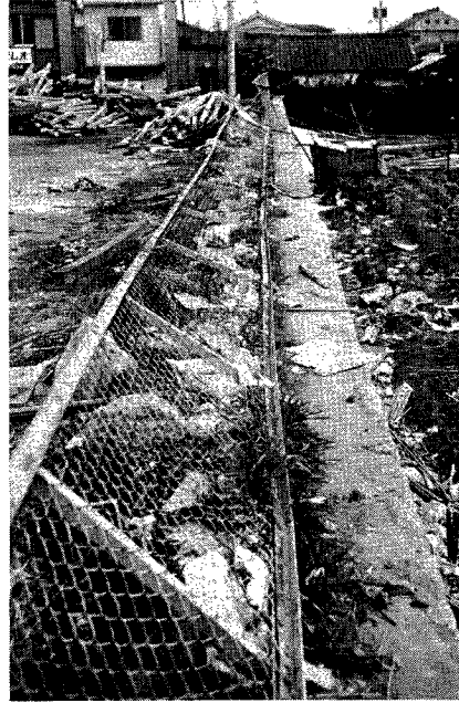
Photo. 6 Damage to a screen fence.
