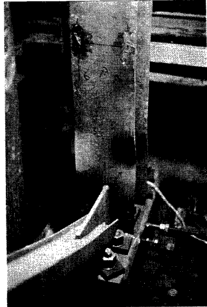
Photo. 9 Local buckling of column bottom (BC5).
