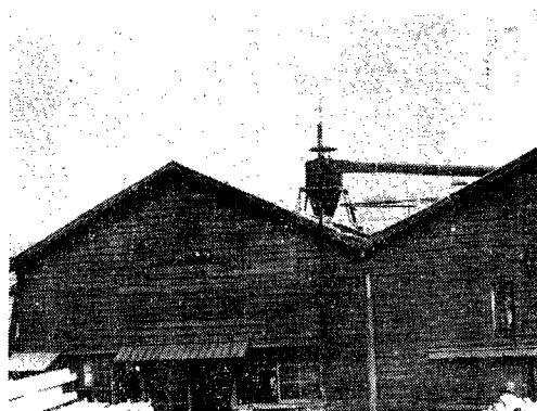
Photo. 1 Separator of saw dust on the roof.
