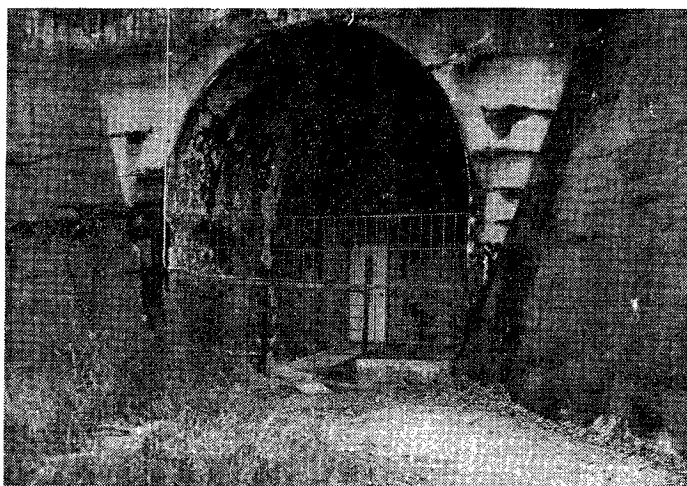
Photo. 1 Entrance of observation tunnel.
