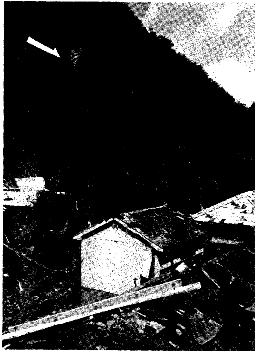
Fig 11. Wind damage to wooden houses in the area shown in Fig10. (by the courtesy of the Shimizu Meteorological Observatory)
