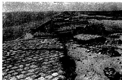
(2) Coastal bank at Mie-prefecture
