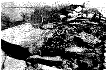
(1) Coastal bank at Aichi-prefecture
