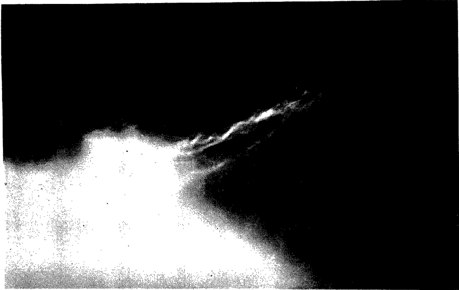
Fig. 12 A radiograph of crack of a reinforced concrete beam (X-ray)
