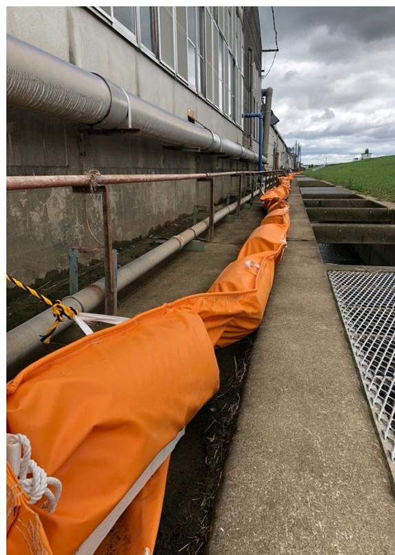
Figure 5. Permanent oil boom implemented in the south side of plant premises, in the closest area to Rokkaku river embankment.
