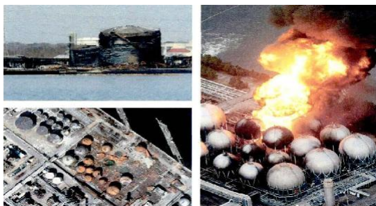
Fig.1 Tank explosion caused by the 2011 earthquake of the Pacificoast of Tōhoku
