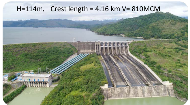
Fig. 6 Photo of the Magat Dam completed on 1982
