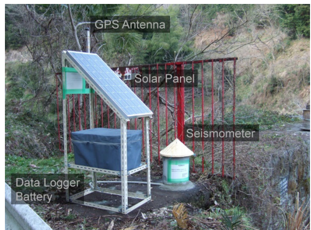
Photo 1. A seismic observation set at Station SL19. The seismometer was placed on a Sabo dam.
