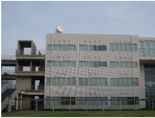
Photo 1 Nagoya University Ka-band polarimetric radar installed at Kobe International University in Rokko Island, Kobe.
