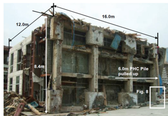
(b) View from the footing side
