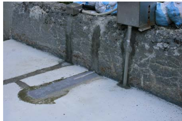
Photo 1 Horizontal and vertical hydrophone set installed in the Ashi-arai dani observation flume
