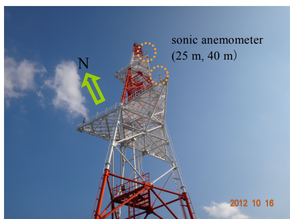
Photo 1 Sonic anemometers on the tower. “N” denotes the direction to the north
