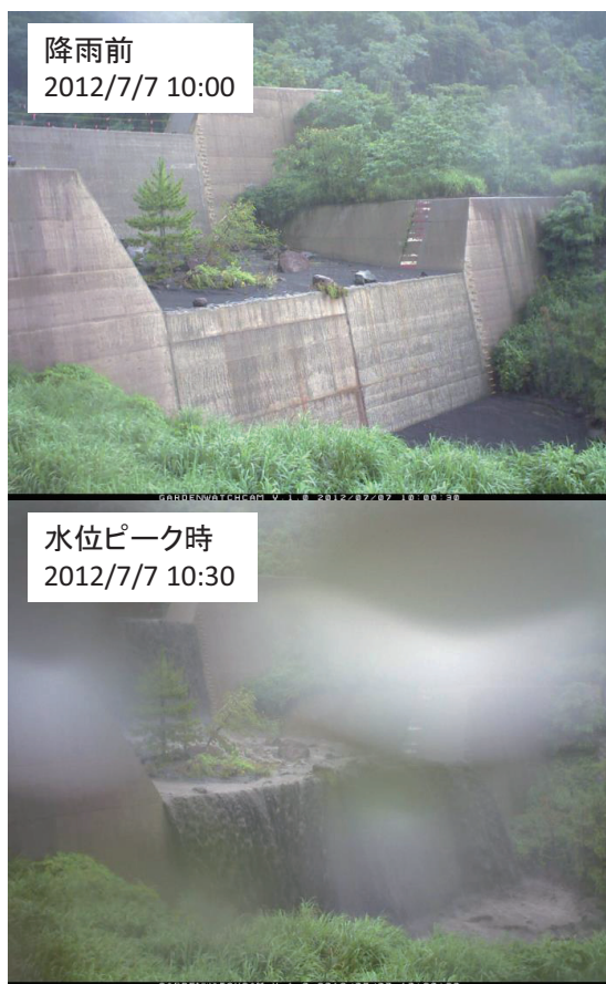
Fig. 7 Stream flow of Furusato River in July 7, 2012
