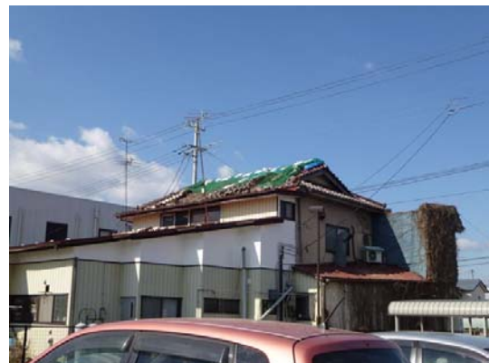
Photo 55 Damage of the roof tiles (site l)
