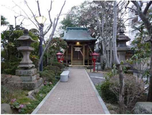
Photo 68 Konpira shrine (after repairing) on 4/18
