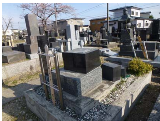
Photo 66 Damage of the graveyard in Zuisen-ji
