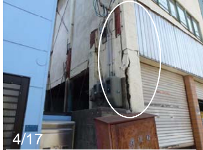
Photo 57 Comparison of the damage of column
