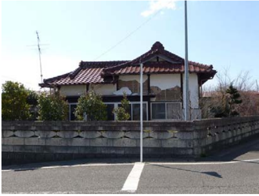
Photo 48 Damage of the plaster wall (site e)
