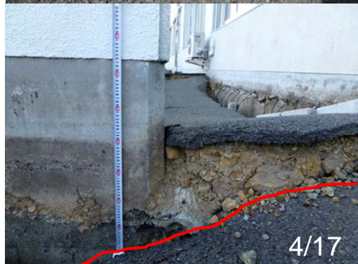
Photo 62 Comparison of the damage of ground pavement
