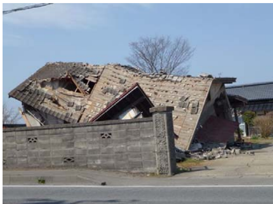
Photo 32 Totally collapsed house in Hirabari area
