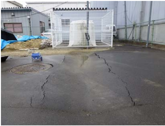
Photo 40 K-NET seismic station in Miyagino fire station
