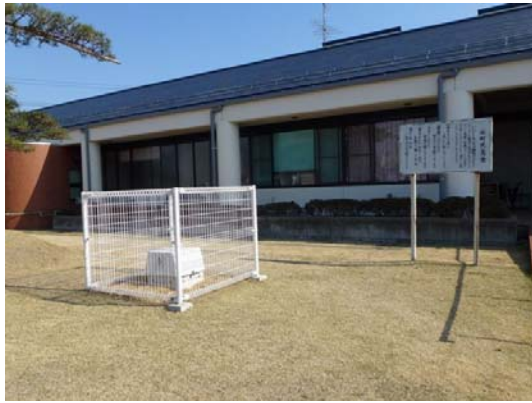
Photo 23 Seismic station at Tome city hall
