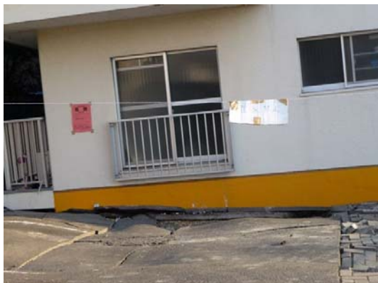
Photo 36 Totally collapsed building in Furukawa area
