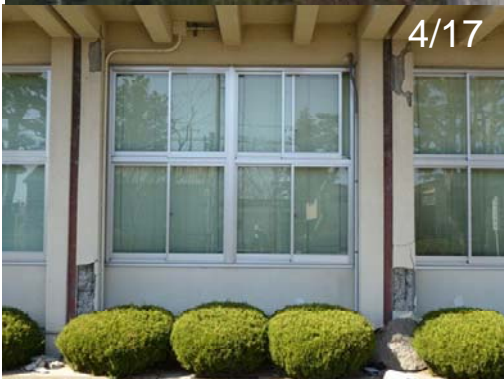
Photo 59 Comparison of the damage of RC column
