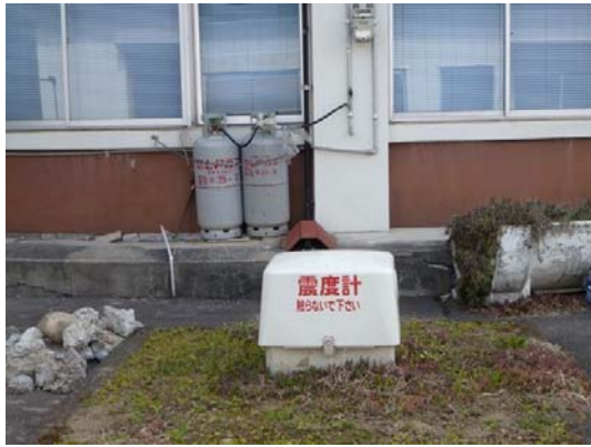
Photo 29 Seismic station at Tajiri branch office
