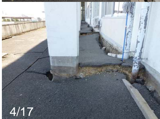
Photo 61 Comparison of the damage of ground pavement
