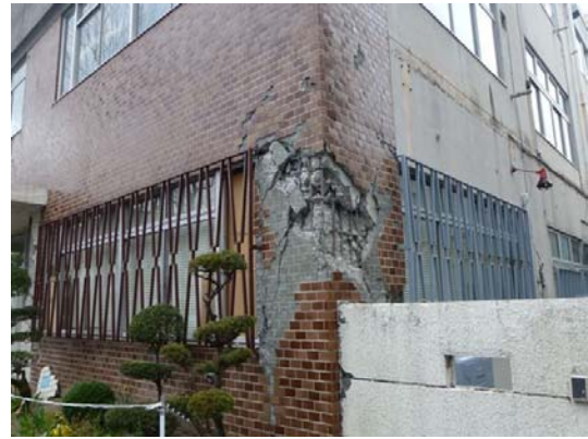
Photo 43 RC column damage in Oroshimachi area
