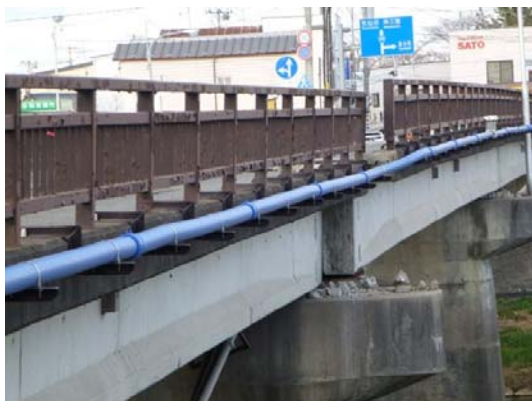
Photo 7 Displacement of Nishiki-bashi
