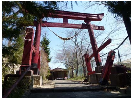
Photo 72 Damage of Tsukidate-Hachiman shrine on 4/17
