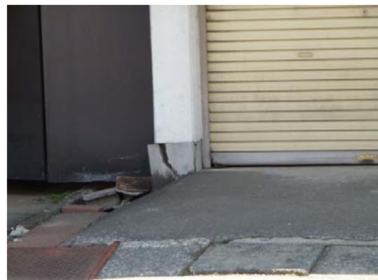
Photo 47 Damage of the foundation (site d)
