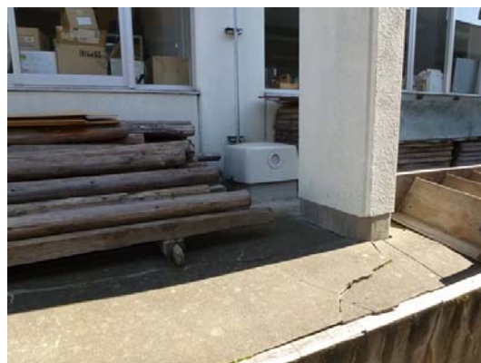
Photo 15 Seismic station at Wakayanagi branch office
