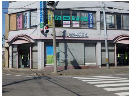
Photo 53 Damage of the glass window (site j)
