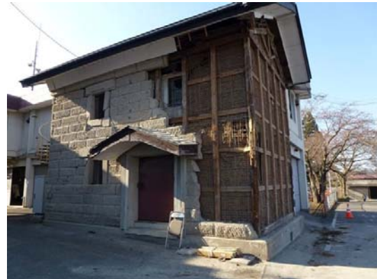
Photo 21 Damage of a storage in Takashimizu area
