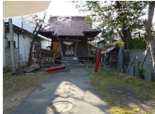
Photo 70 Damage of Nishinomiya shrine on 4/18
