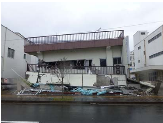
Photo 42 Totally collapsed building in Oroshimachi area
