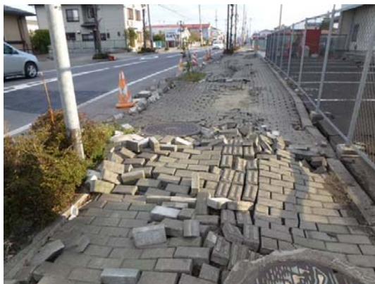
Photo 6 Ground damage in Sanuma area
