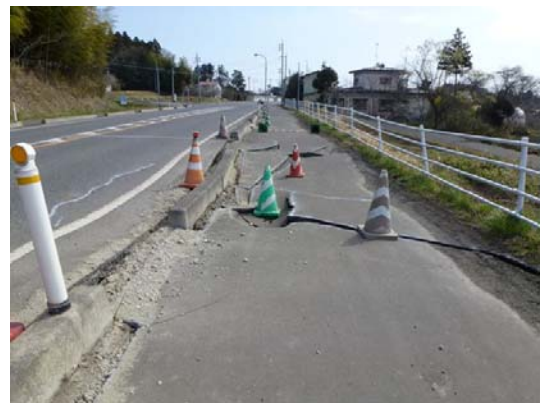
Photo 27 Ground damage along the prefecture route 1
