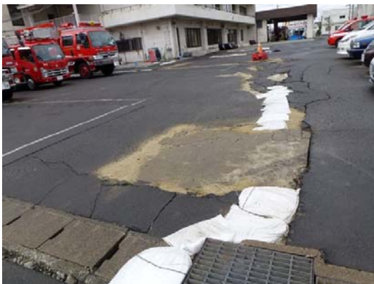
Photo 41 Ground damage at Miyagino fire station
