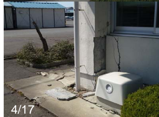
Photo 60 Comparison of the damage at the seismometer
