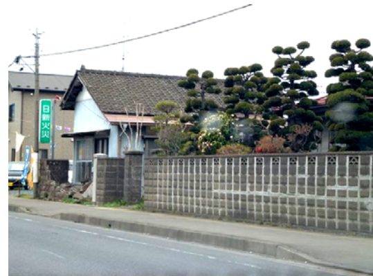
Photo 39 Damage of the concrete block wall
