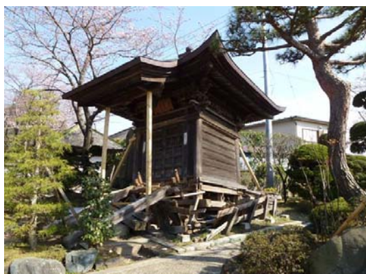
Photo 65 Damage of the building in Zuisen-ji
