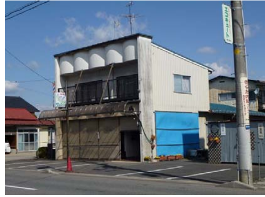
Photo 52 Damage of the exterior wall (site i)
