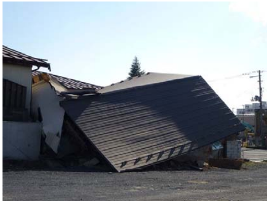
Photo 5 Totally collapsed house in Sanuma area
