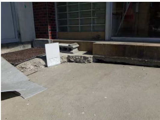
Photo 50 Damage of the foundation (site g)
