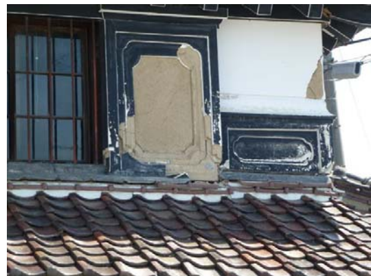
Photo 46 Damage of the plaster wall (site c)
