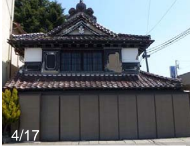
Photo 56 Comparison of the damage of plaster wall
