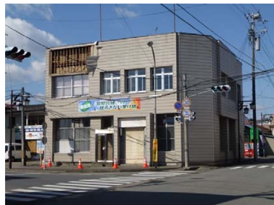
Photo 10 Damage of the wall in Tsukidate area
