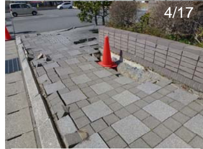
Photo 58 Comparison of the damage of ground pavement
