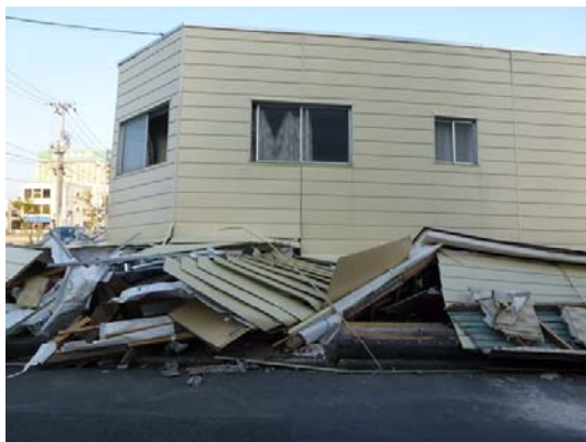
Photo 35 Totally collapsed building in Furukawa area
