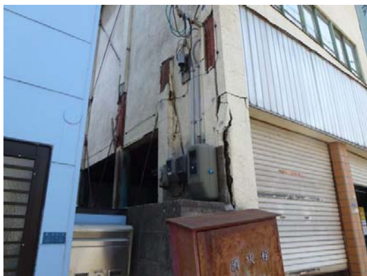
Photo 45 Damage of the exterior panel (site b)
