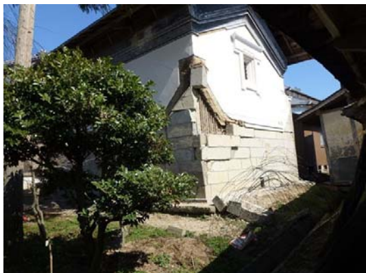
Photo 13 Damage of a storage in Shiwahime area
