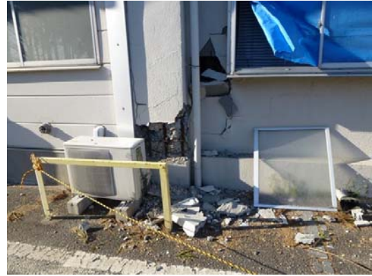
Photo 20 Column damage of Takashimizu branch office
