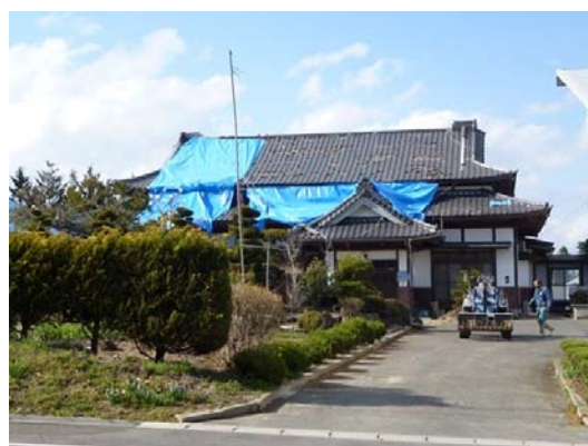
Photo 4 Damae of the roof tiles in Naganuma area
