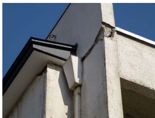
Photo 3 Building damage of Semine branch office
