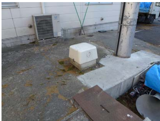
Photo 19 Seismic station at Takashimizu branch office
