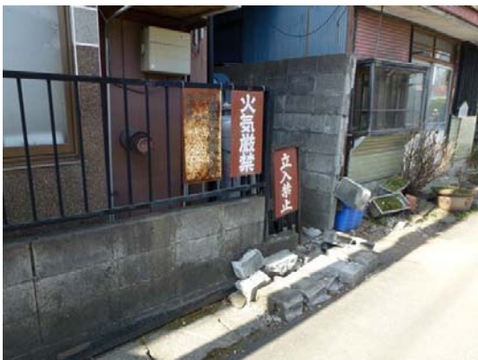
Photo 51 Damage of the concrete block wall (site h)
