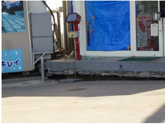
Photo 17 Ground damage in Wakayanagi area
