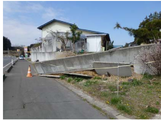
Photo 26 Ground damage along the prefecture route 1
