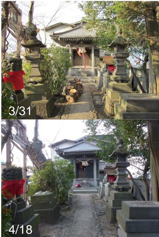
Photo 69 Damage of Kanaya shrine (3/31 and 4/18)
