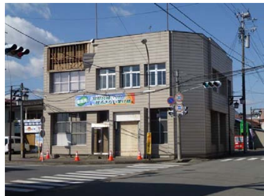
Photo 54 Damage of the exterior panel (site k)
