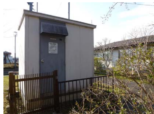
Photo 33 JMA seismic station in Furukawa area
