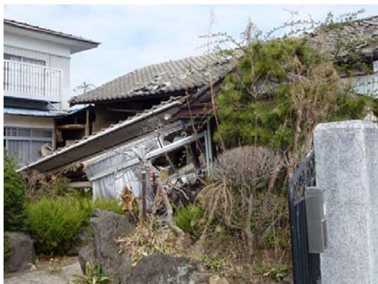
Photo 31 Totally collapsed house in Tajiri area
