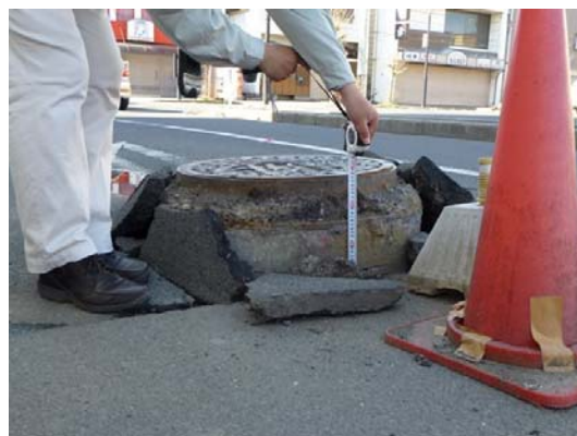
Photo 16 Floating of a manhole in Wakayanagi area
