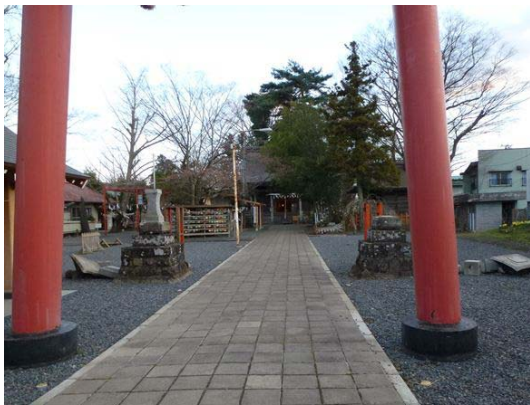
Photo 71 Damage of Tsushima shrine on 4/16
