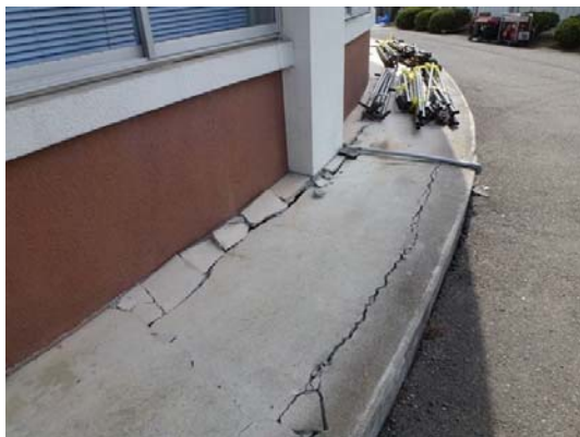
Photo 30 Base damage of the Tajiri branch office
