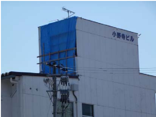
Photo 49 Damage of the exterior panel (site f)
