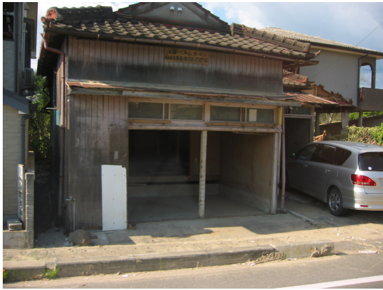
Fig. 6 Damaged house in the Torai area
