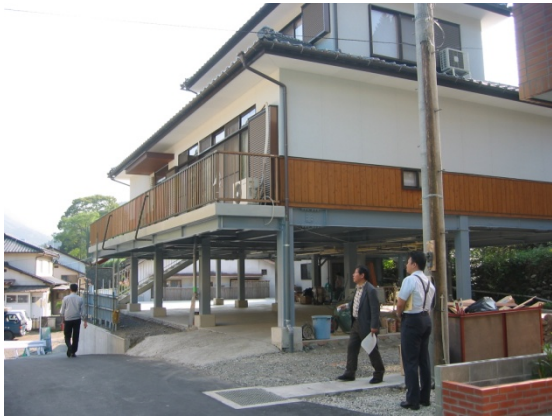
Fig. 9 A house that completed raising its floor
