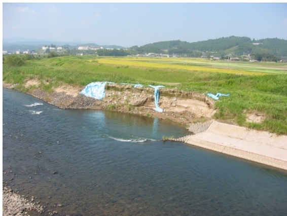
Fig. 7 Eroded river bank
