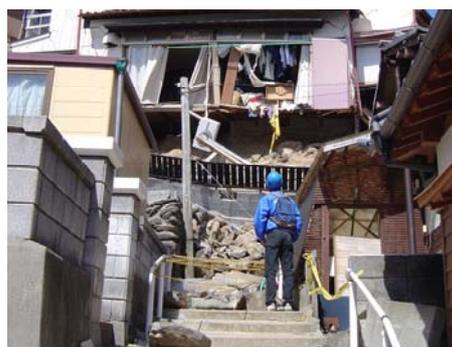
Photo.2 Typical damage of wooden house
