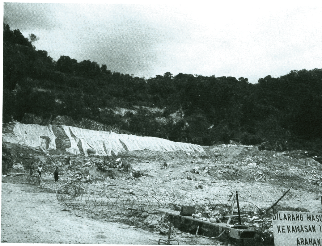
Photo 9 Site of collapsed building, fortnight after toppling.
