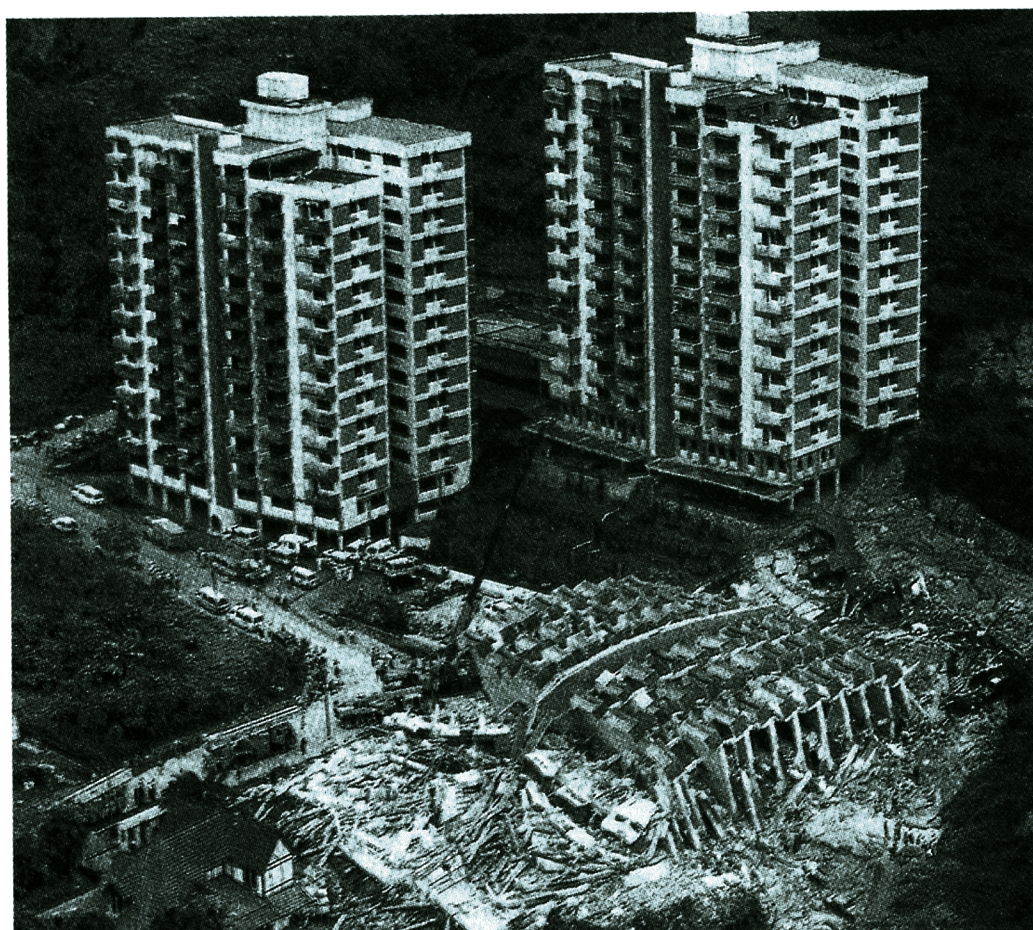
Fig. 4 Copied picture of Highland Towers disaster. (New Straits Times, Dec. 13, 1993)
