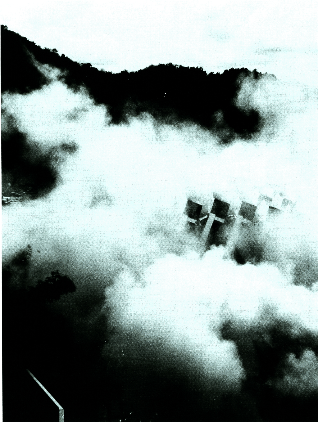
Photo 6 Smoke of the building, 3 minutes after toppling.
