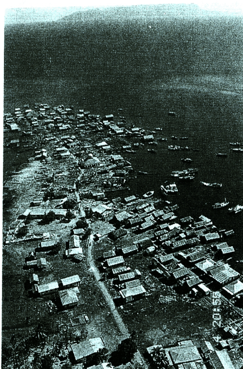
Photo 1 Aerial view of Wuring village damaged by tsunamis.
