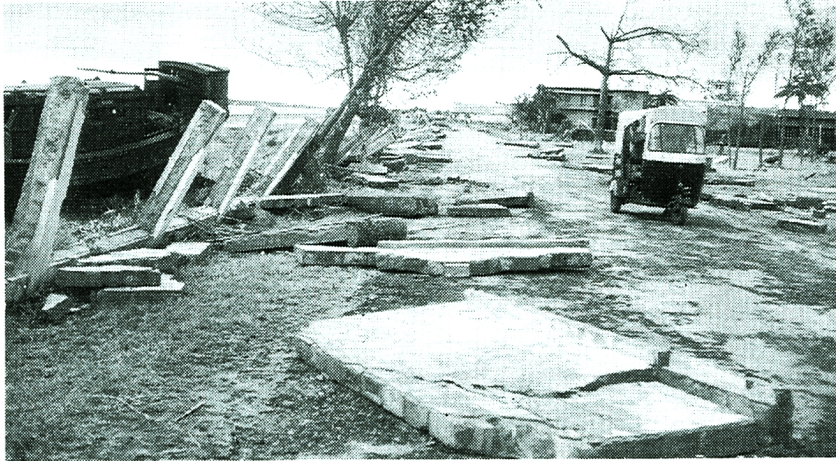
Photo 6. Brick wall toppled by flooding water.
