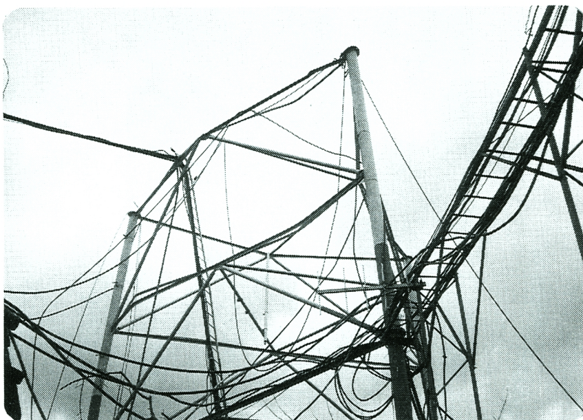
Photo 5. Destruction of an antenna tower. Photograph taken by Mr. H. Baba, 1st Secretary of the Embassy of Japan.
