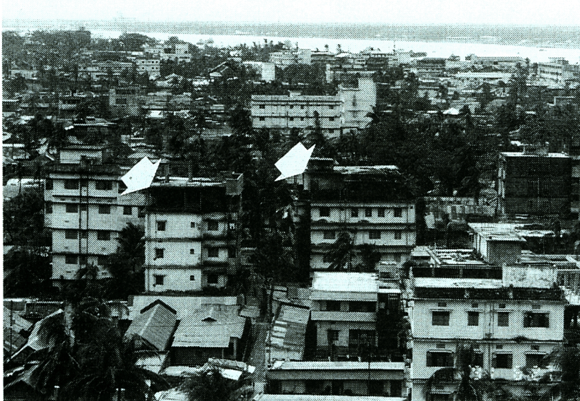
Photo 2. Blowdown brick walls.
