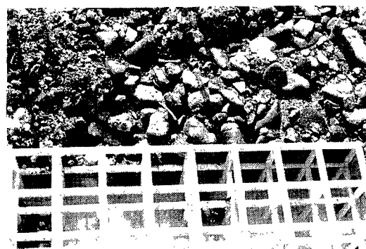
Photo. 2 Inter-locking feature of sediment particles in the square grid dam.
