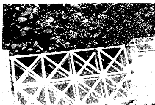
Photo. 1 Inter-locking feature of sediment particles in the zigzag grid dam.
