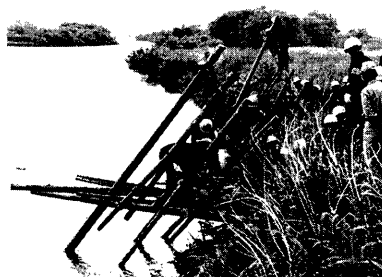
Photo 2 Kawakura in the Jintsu River (during a flood fighting drill)
