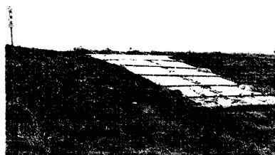
Photo 4 Harinuno-ko (cloth mat covering) in the Yodo River (during a flood fighting drill)
