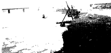
Photo 1 Kawakura (a kind of wooden framed jetty) in the Joganji River (during a flood)
