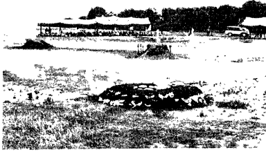
Photo 7 Kamadan ko (circular hooping by sandbags) in the Yodo River (during a flood fighting drill)
