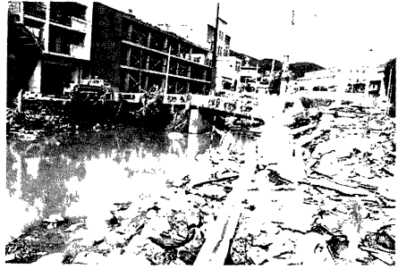
Photo. 3 An example of disaster caused by flash flood: Stream banks were eroded, and pipe line was injured.
