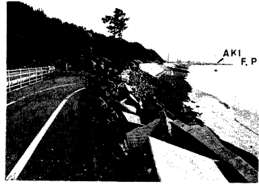
Photo.3 Breakdown of seawalls caused by Typhoons 7916 and 7920 at Aki Nishihama coast.
