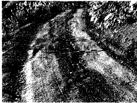
Photo 2. A surface pattern of a unpaved road.
