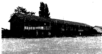
Photo. 3. Damage of roof of timber structures (Minamikoizumi primary school).
