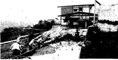
Photo. 17. Failure of slope.
