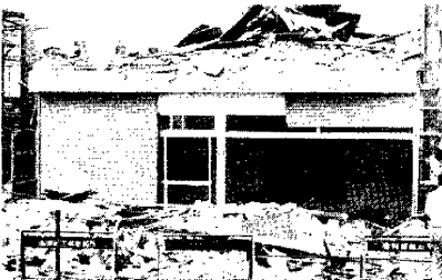
Photo. 28. Damage of C-structure.
