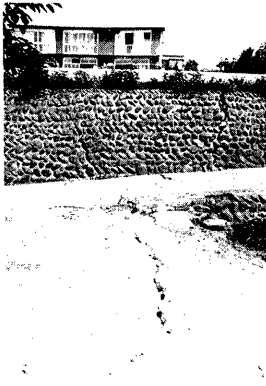
Photo. 19. Failure of slope and damage of retaining wall.
