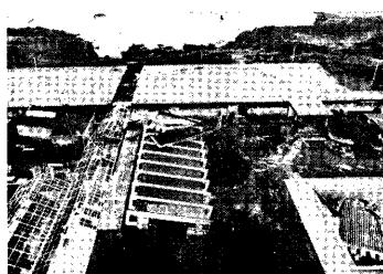
Photo. 10. Damage to cement tile roof: steel frame.
