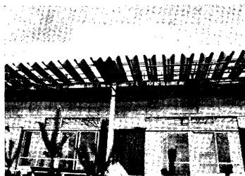
Photo. 11. Damage to roof: steel frame.
