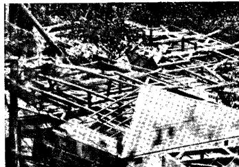
Photo. 4. Roof failure due to uplift: wooden house.
