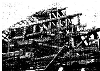
Photo. 6. Roof failure due to uplift: traditional house.
