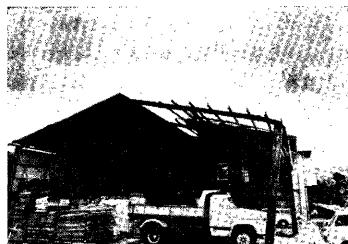
Photo. 13. Damage to steel frame: warehouse.
