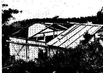
Photo. 14. Damage to temporary house: light steel frame.
