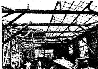
Photo. 2. Roof failure due to uplift: warehouse.
