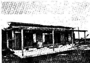
Photo. 1. Roof failure due to uplift: wooden house.
