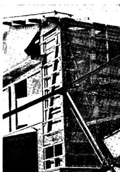
Photo. 3. Damage to external wall: wooden house.
