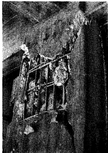
Photo. 9 Hachinohe City Office Building
