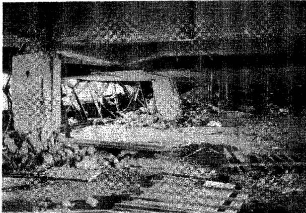
Photo. 2 Mutsu City Office Building
