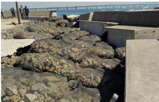
Fig.1 PU applied in Kansai International Airport
