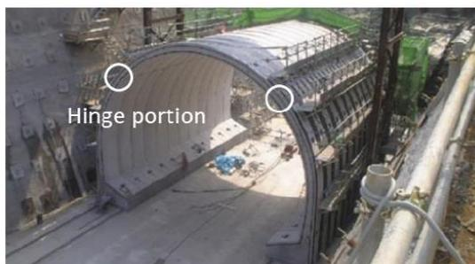
Photo 1. Single unit two-hinge precast arch culvert
