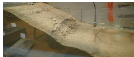
Fig. 7. Damage to embankment after rapid drawdown
