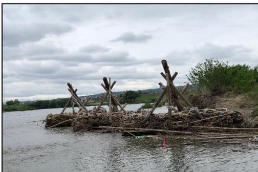
**Fig. 1** Seigyu structure located at the right bank of Kizu River
