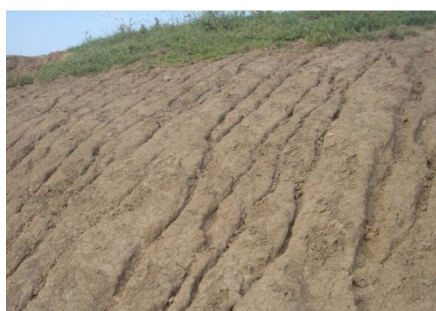
Fig.1 The slope before modification
