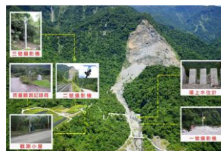
Figure 1 Landslide dam monitoring system
