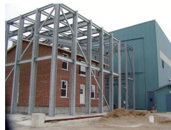
Figure 3: Full scale wind vulnerability testing
