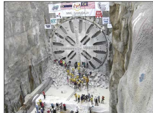
Tunnel Boring Machine broke through at South Junction Box on 04/06/05
