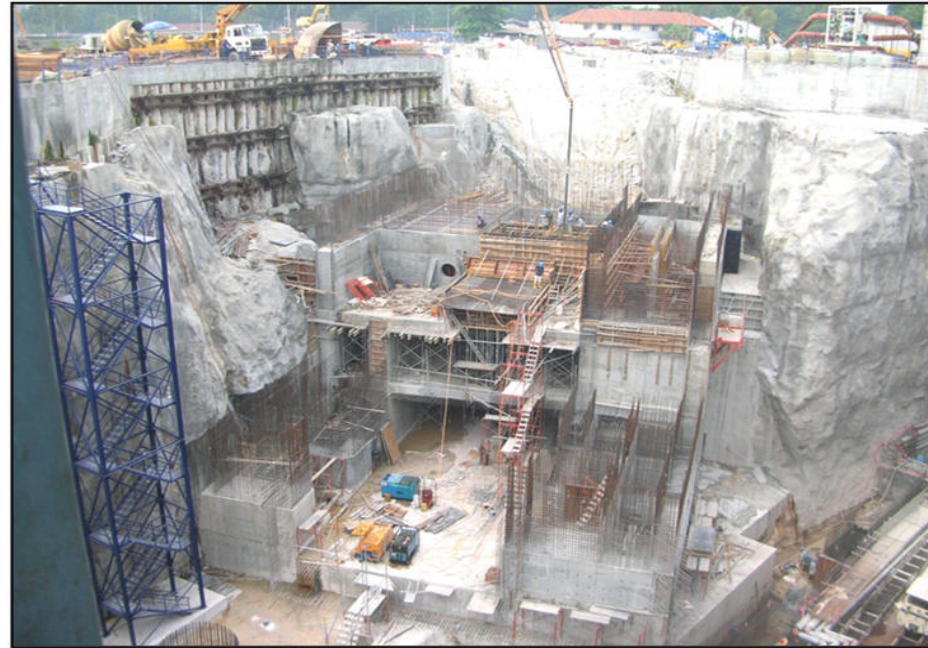
Vent shaft structural works in progress
