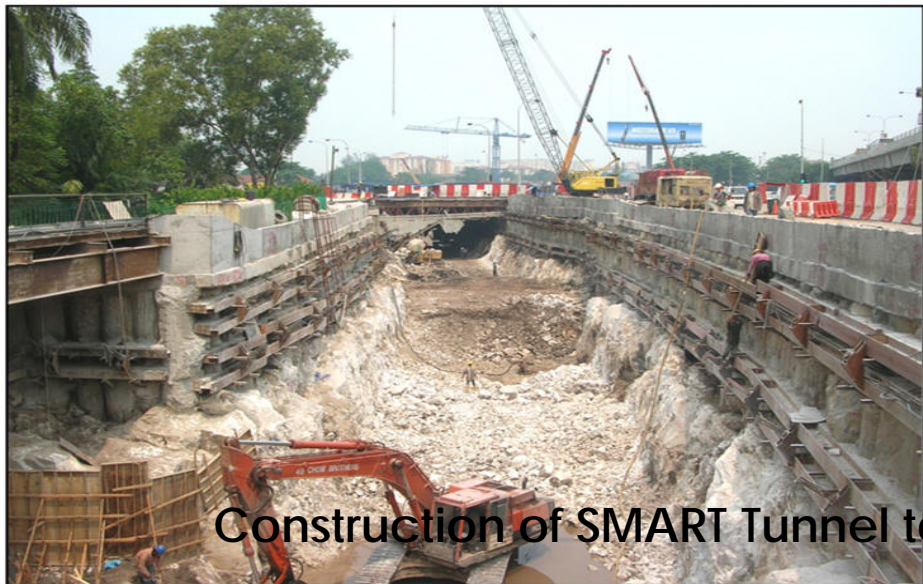
Rock excavation at Jalan Tun Razak MN03 in progress
